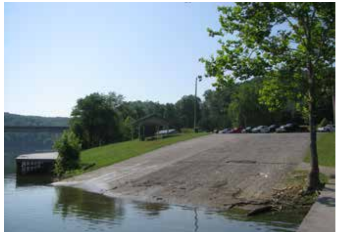
The large boat ramp needs resurfacing.
