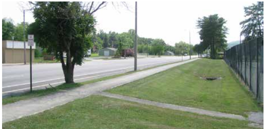
The connector paths are very narrow and not ADA compliant.
